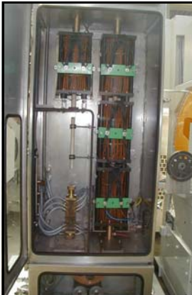
Inductor coil arrangement
